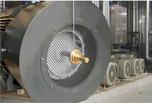
Patented SGS™ CL Series Shaft Grounding System
